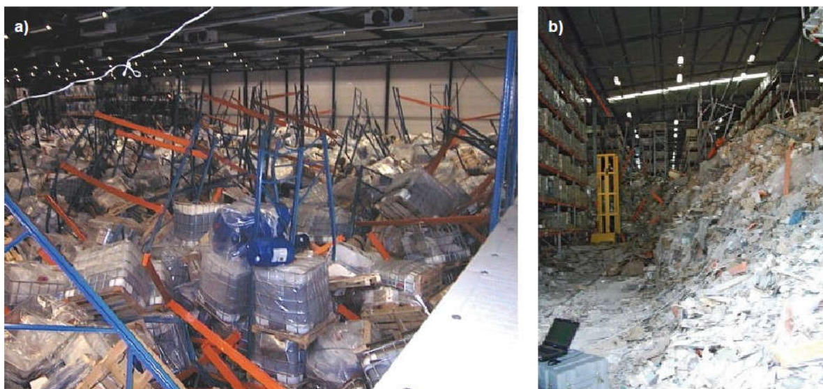
Figure 1: A minor collision can result in total collapse due to the dynamics of pallets falling
