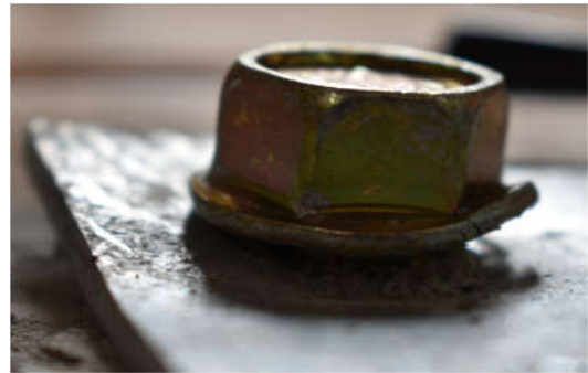
(b) Bolt loosened & pulled out a little
