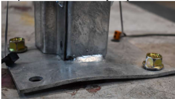
(a) Ductile baseplate permanent deformed
