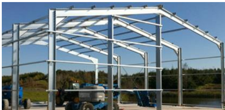
Figure 1: Photograph of a CFS portal frame building.
